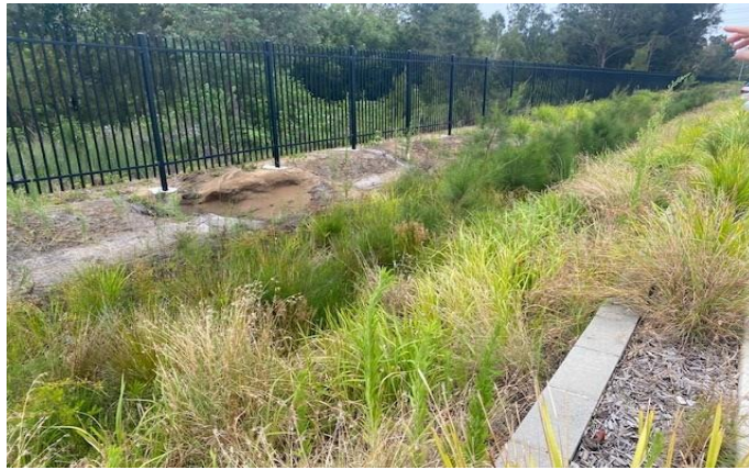
Photo 9: Minor scour of drainage line along west boundary
