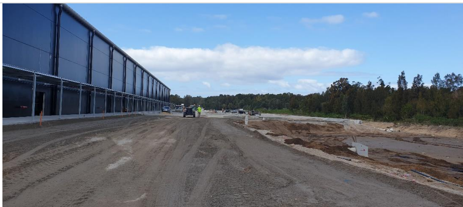
Photo 9 – Taken 2 September 2020 – backfilling of the parking area at the western portion of the site.
