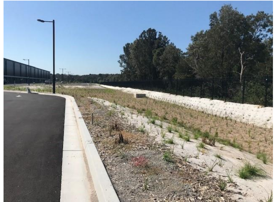
Photo 4 – taken on 18 January 2021 - Permanent fencing and swale installed along the site perimeter. Photo taken at the western perimeter.
