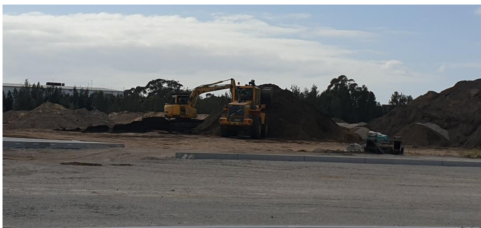
Photo 9 – Taken 2 September 2020 – backfilling of the parking area at the western portion of the site.
