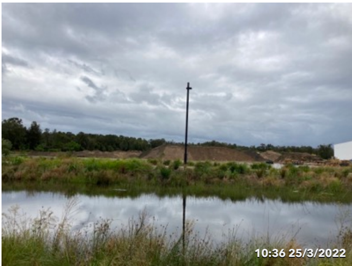
Photo 20 Stage 2 Warehouse area
