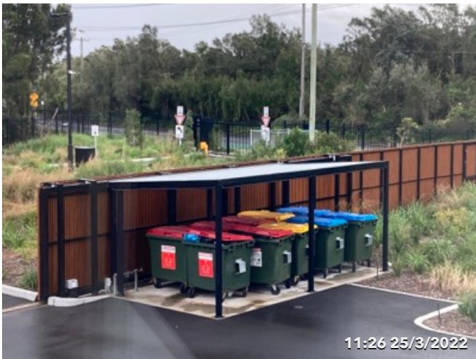
Photo 64 Waste truck collection area
