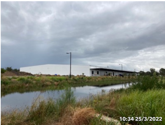
Photo 17 Stormwater swale at the eastern perimeter
