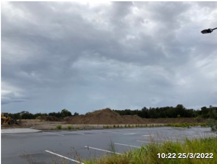
Photo 9 Stage 2 Warehouse Cleanup works segregating materials and grading
