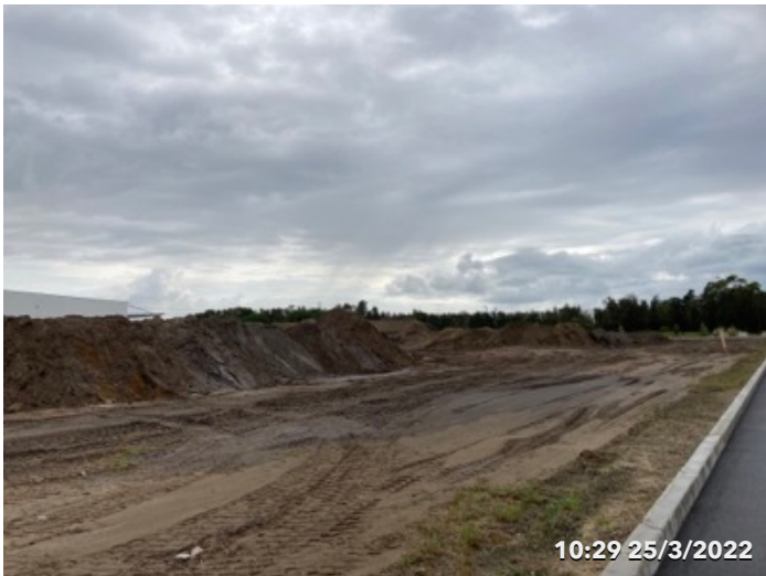
Photo 12 Stage 2 Warehouse area clearing and grading
