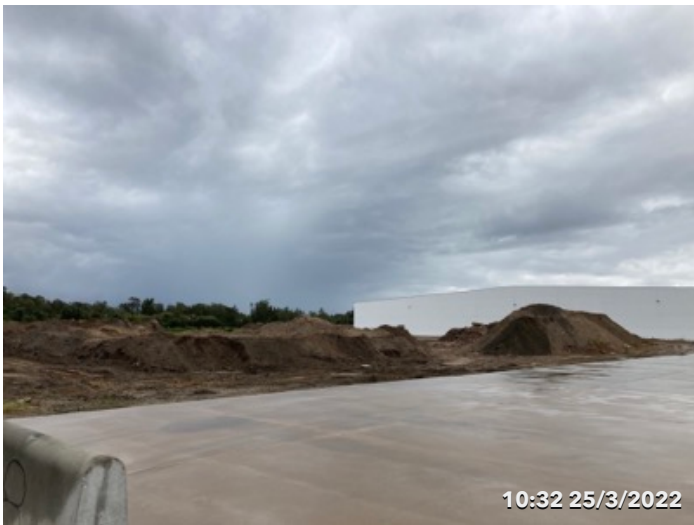
Photo 14 Stage 2 Warehouse area
