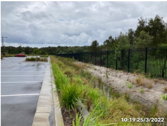
Photo 8 Swale along the west perimeter
