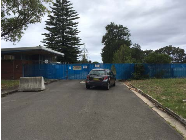
Picture 1: Main Entry from Captain Cook Drive
