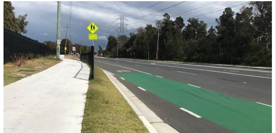
Photo 24 – Taken from bus stop showing marked cycle lane and pedestrian refuge adjacent to site perimeter fencing
