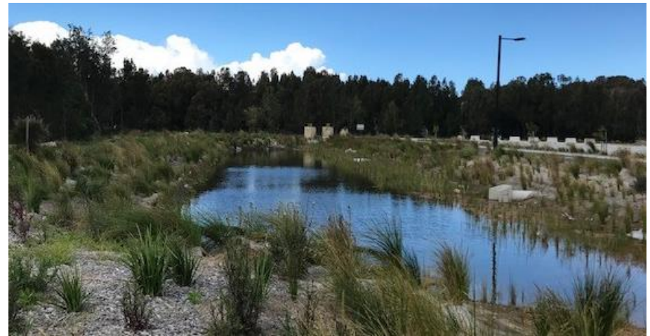
Photo 14 – Water catchment area
