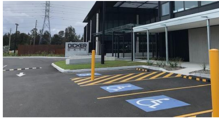
Photo 20 – Disabled parking bays accessible to main entrance
