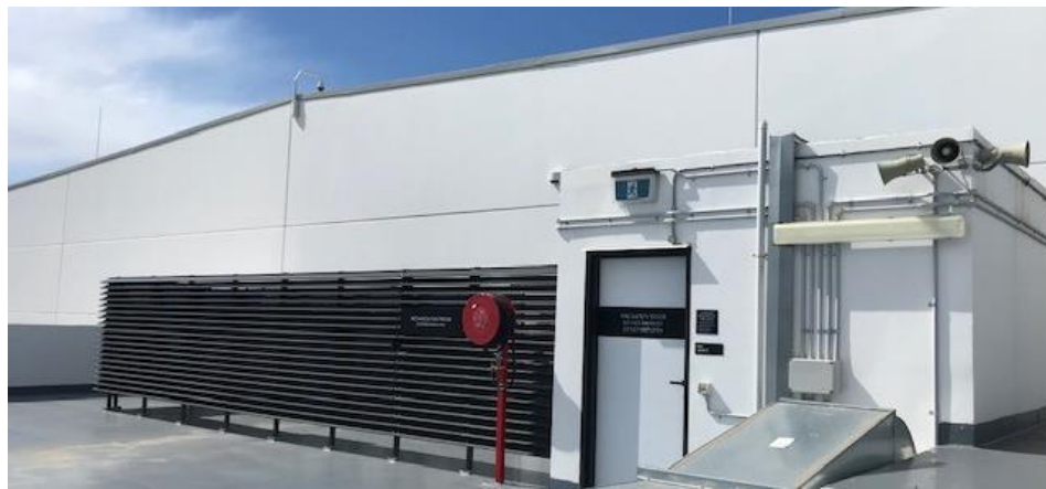
Photo 21 – Implemented fire safety measures as recommended
