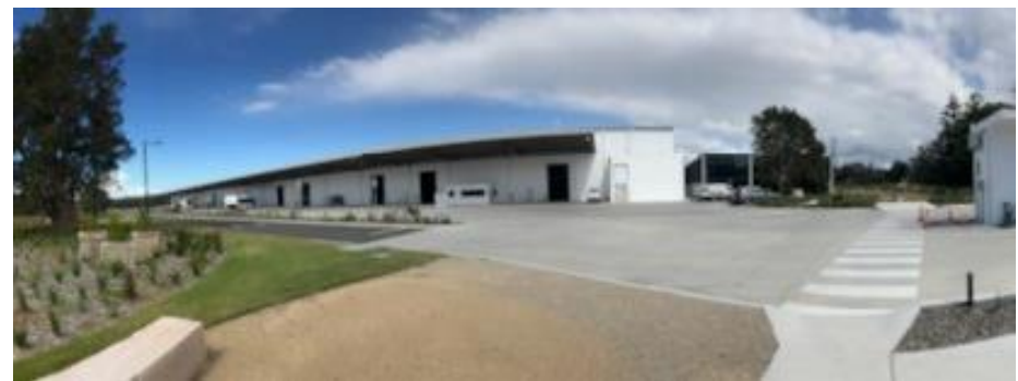
Photo 4 – Panoramic view of warehouse exterior taken from delivery gate
