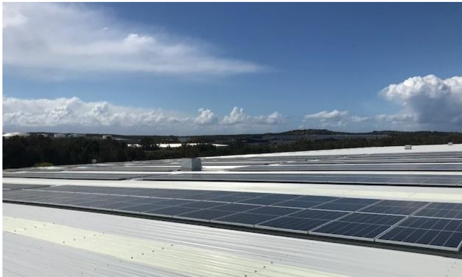
Photo 1 – Solar panels installed
